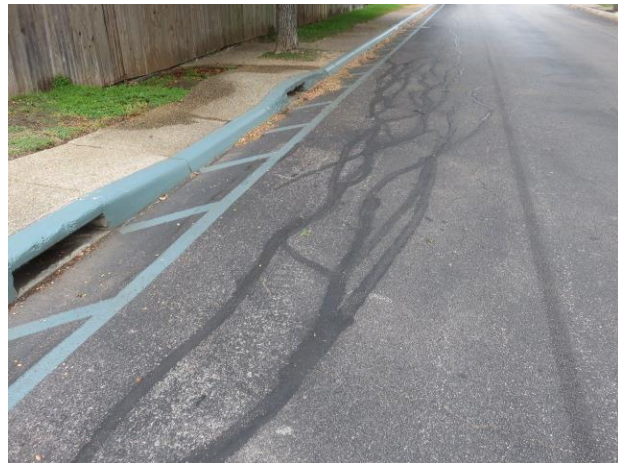
Repaired edge cracks
