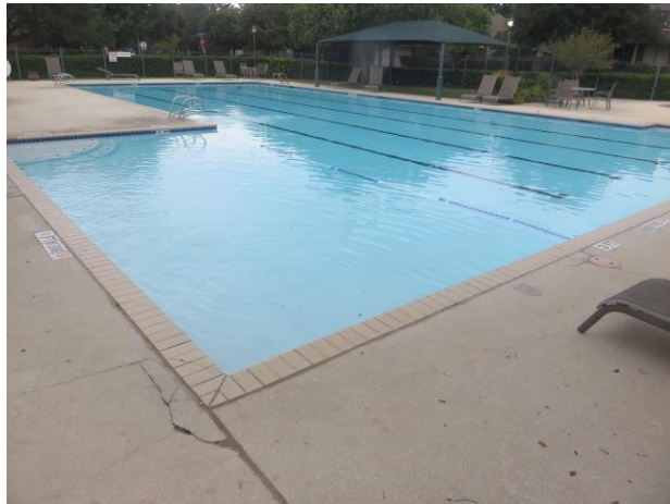
Pool structure with plaster pool finish
