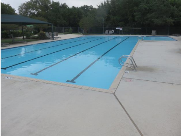
Pool and deck overview
