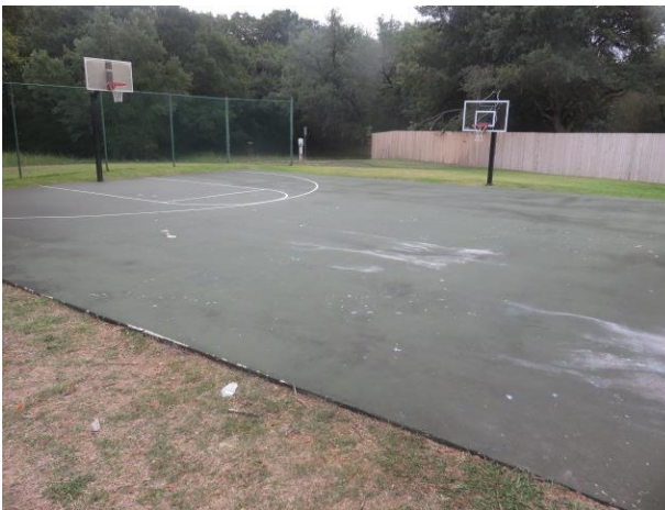
Basketball court overview
