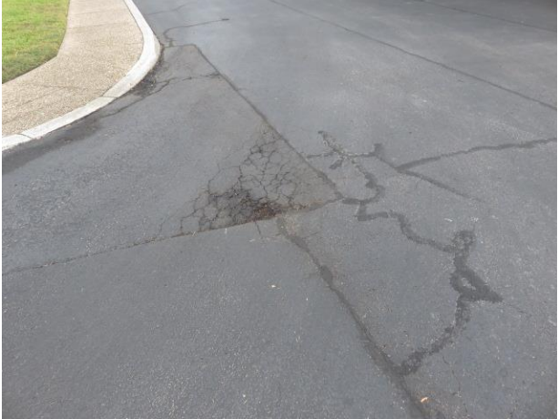
Pavement deterioration
