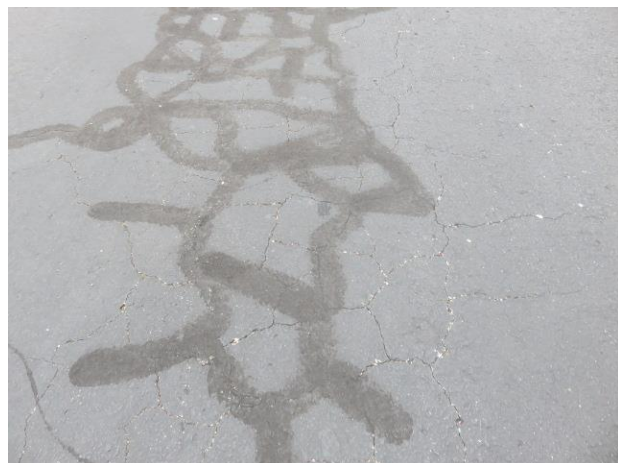
High frequency of cracks
