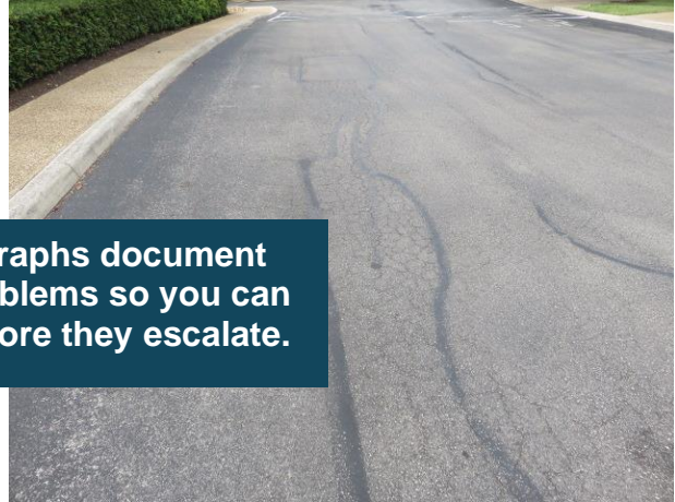
Alligator cracks
