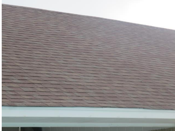
Dimensional asphalt shingle roof assembly in good condition
