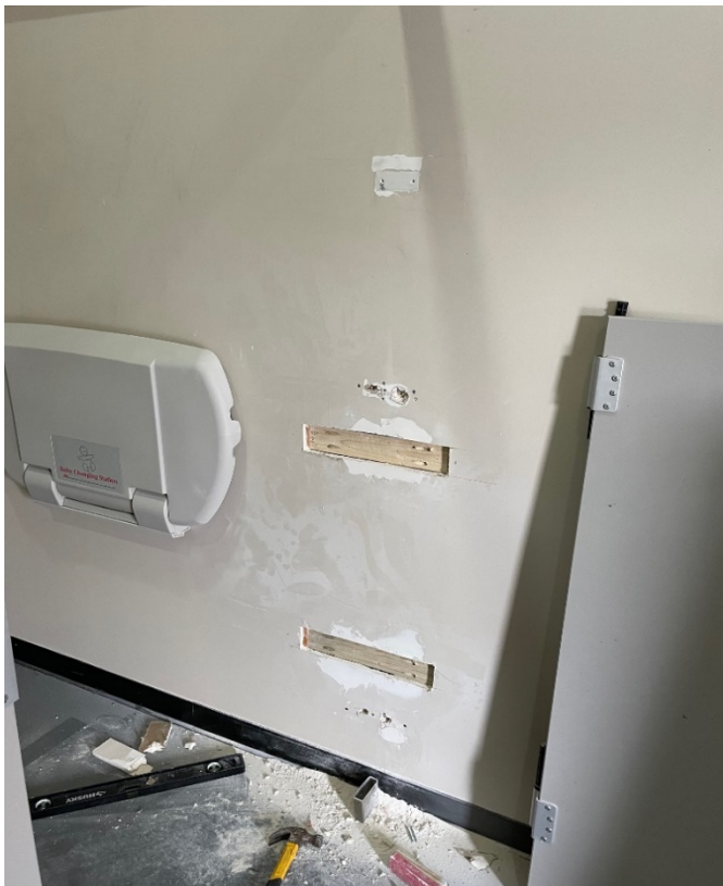
Repaired holes in sheetrock
