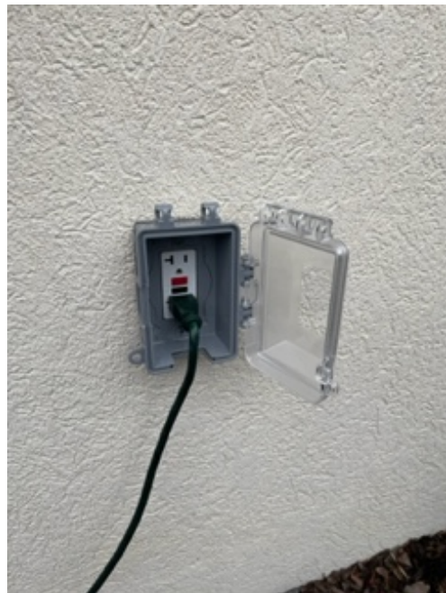
Installed a new electrical outlet & cover.
