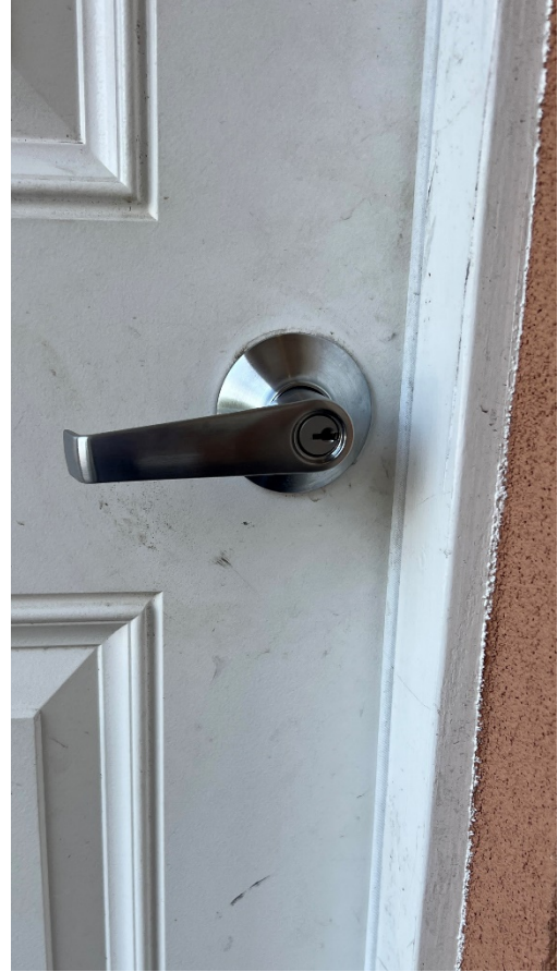
New commercial grade door handles have been installed.
