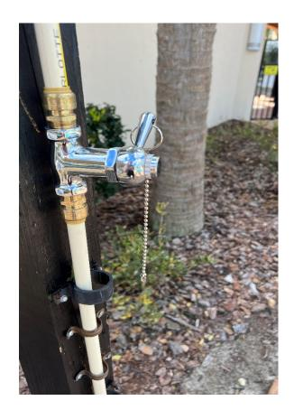
Outside pool shower pipe has been replaced and has a new valve.
